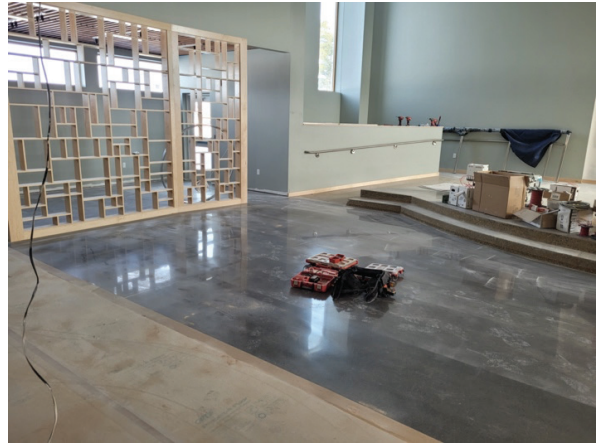
View from Sanctuary showing the west chapel
